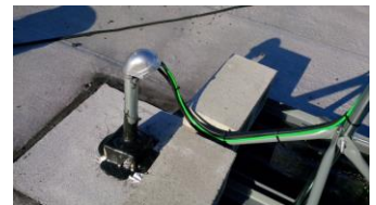
sent into the building ...
